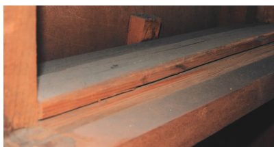
Photo 8. Wedge inside chest to support thin side panel. AP
